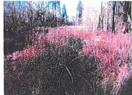
Power Line Right-of-way
