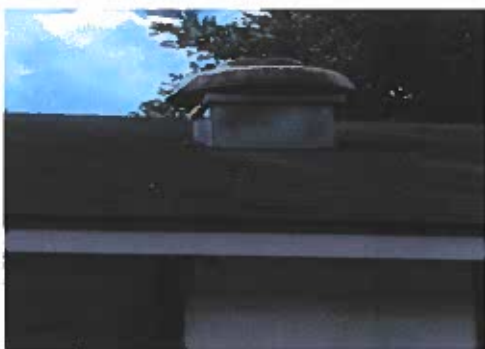
Top left exhaust vent
